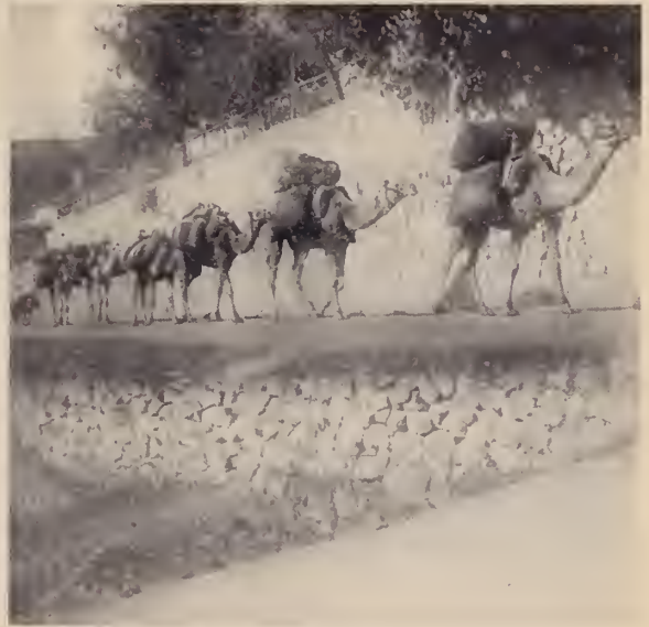
LINKED CAMELS UNDER THE YARD WALL OF ZAHLEH MANSE.
